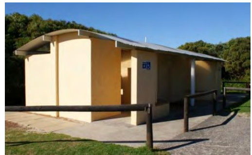
Public toilets at Peaceful Bay (second car park)
