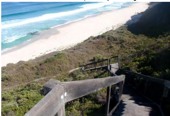
Pedestrian access timber staircase at Back Beach
