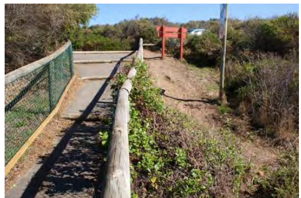
Pathway extending from Ocean Beach Lookout car park down the cliff
