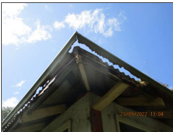
Damaged gutters
