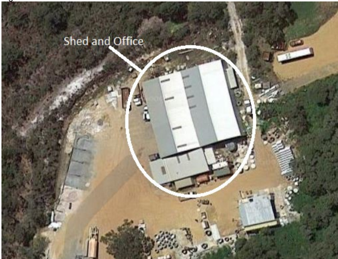
Aerial image from Google Maps
