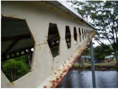
RBN – Roof Beam North
