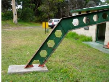
North east Elevation – Pad footing PFN, to Roof beam RBN
