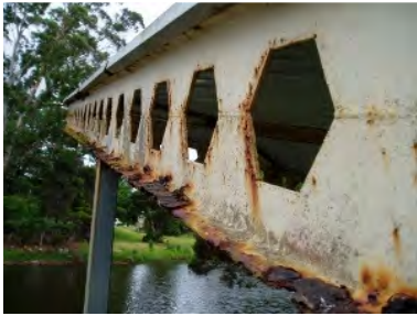
RBS – Roof Beam South
