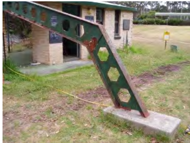
South east Elevation – Pad footing PFS, to Roof beam - RBS
