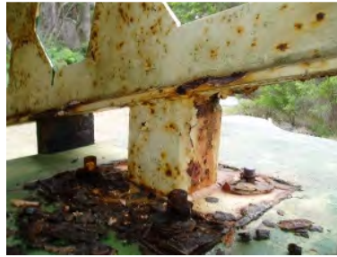
SCS – Stub columns South
