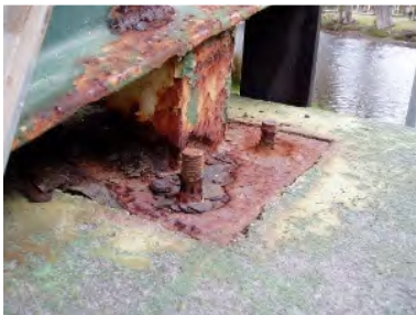
SCN – Stub columns North [eastern view]
