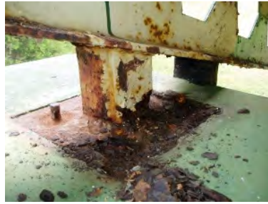
SCN – Stub columns North [western view]
