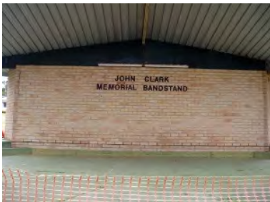
West Elevation - brickwork
