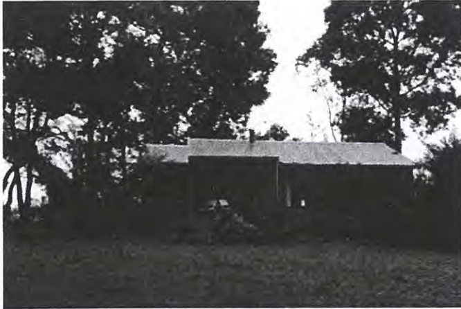
One of two current existing chalets
